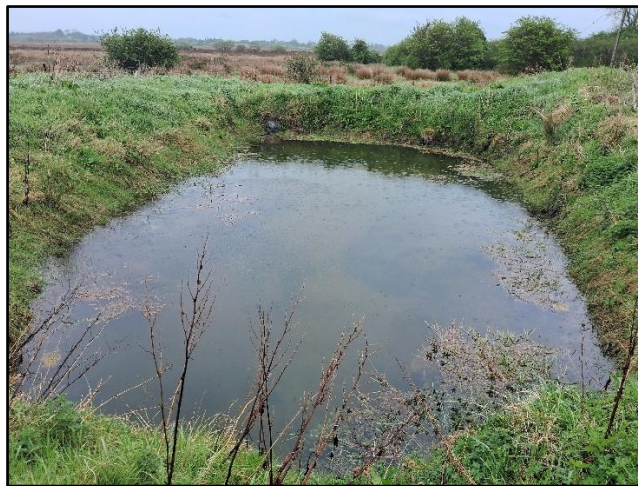
Figure 9: Existing excavation and pond on the site (image taken on 24/04/2025).
